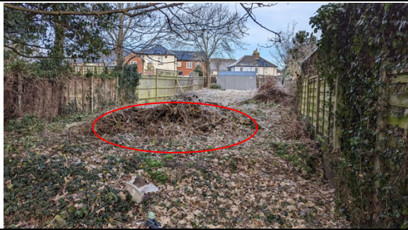
Photograph 3 – Looking north with a pile of old concrete rubble in the middle of the plot (red circle).
