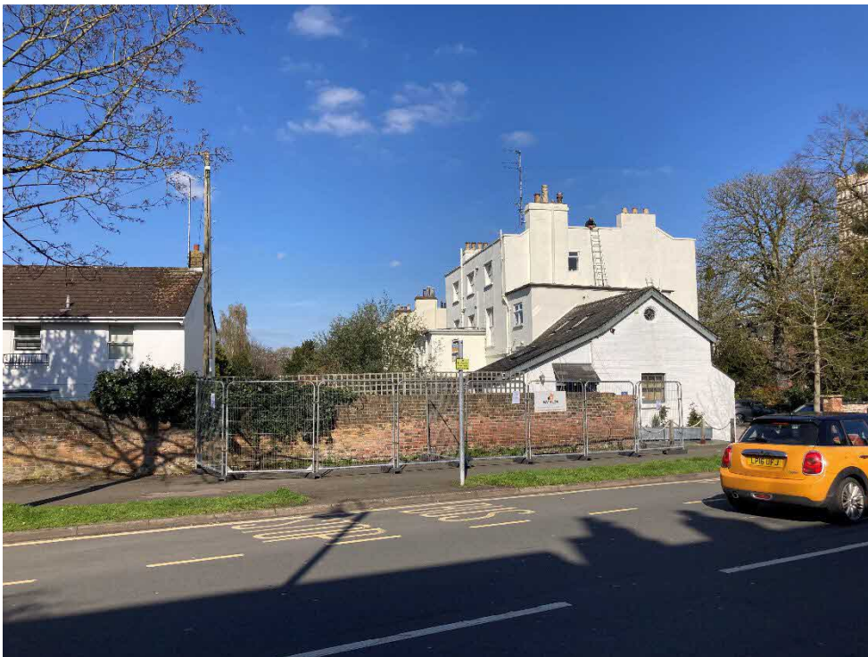
ii. Location of unsafe wall
