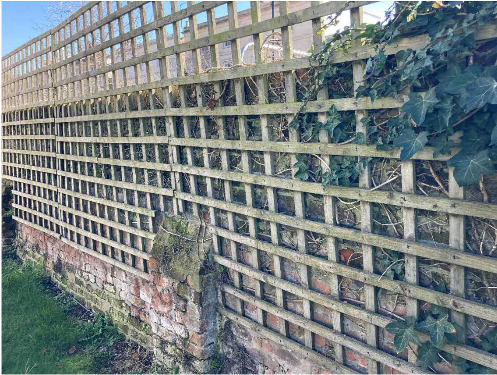
XIX. Crack running vertically through buttress. XX.
