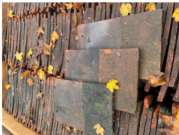
Fig 4. ROOF: Reclaimed clay tiles
