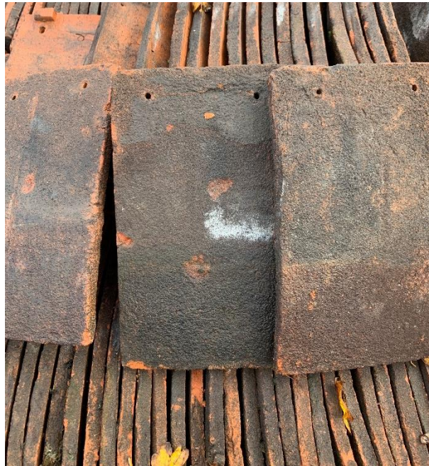
Fig 5. ROOF: Reclaimed clay tiles
