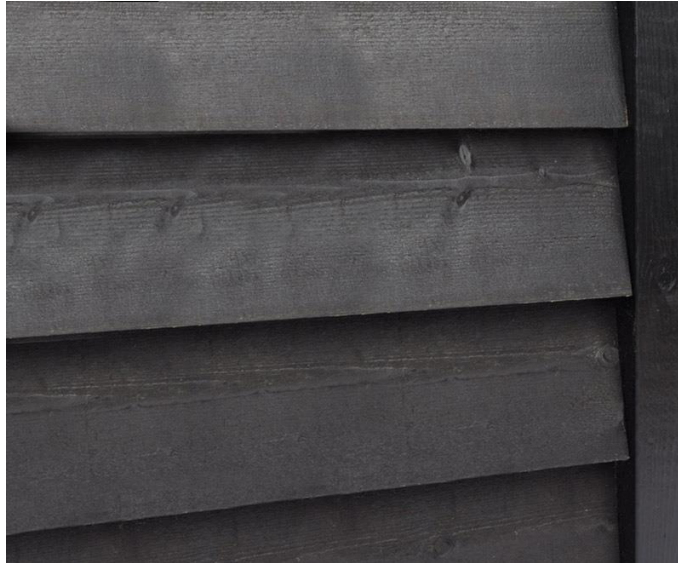
Fig 2. WALLS: Horizontal timber cladding (featheredged), painted black
