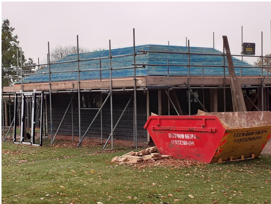
Fig10. As-Built Outbuilding as per 16 th November 2023, viewed from within the site
