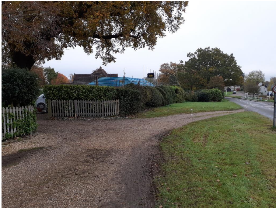
Fig8. As-Built Outbuilding as per 16 th November 2023, viewed from The Green
