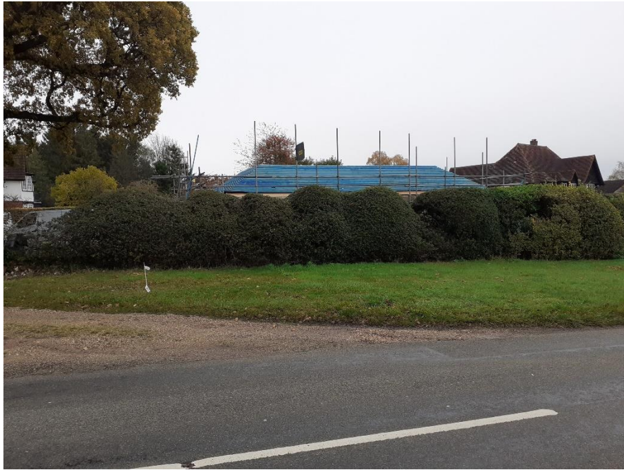
Fig7. As-Built Outbuilding as per 16 th November 2023, viewed from The Green
