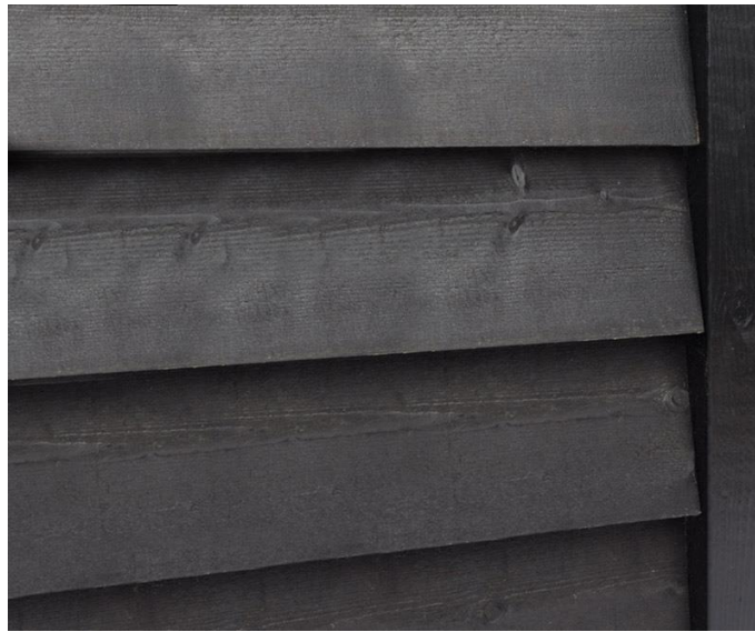
Fig 11. WALLS: Horizontal timber cladding (featheredged), painted black
