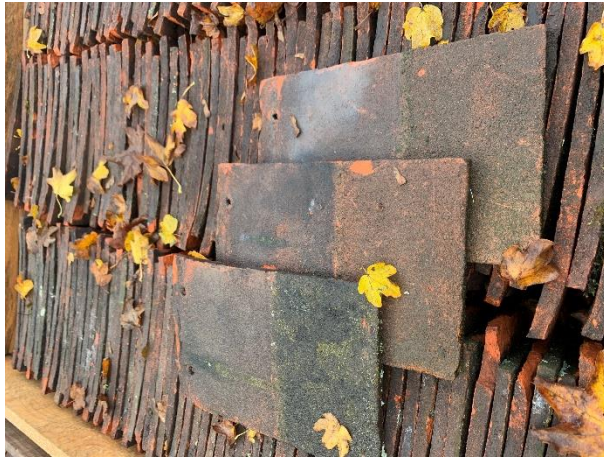
Fig 13. ROOF: Reclaimed clay tiles
