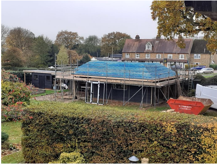
Fig9. As-Built Outbuilding as per 16 th November 2023, viewed from within the site
