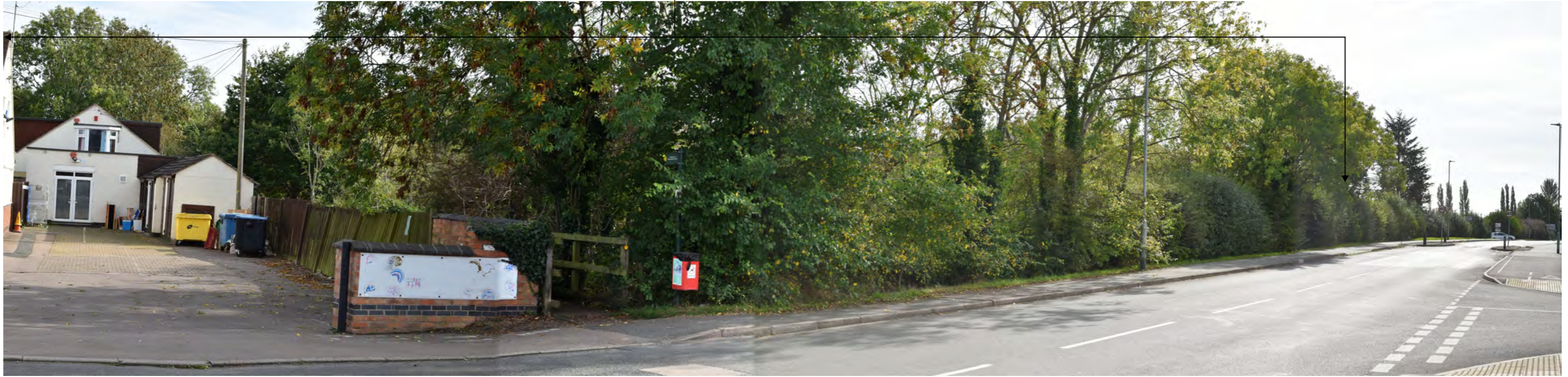
View 1 - From Lutterworth Road approximately 15m from the site looking south-east
