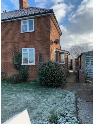
View of house, garage, hardstanding, ornamental shrubs, and amenity grassland from the road.
