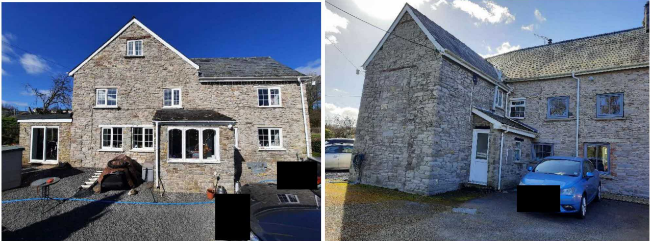
Plate 3: Showing the southeast gable and elevation. Plate 4: Northeast gable and northwest elevation.
