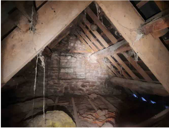
Plate 9: Loft of northeast extension. Looking northeast to gable end.
