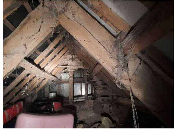
Plate 10: Looking southwest towards join with main house roof.
