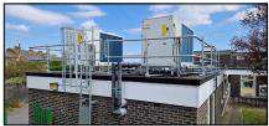
Typical Rooftop ASHP & Enclosure
