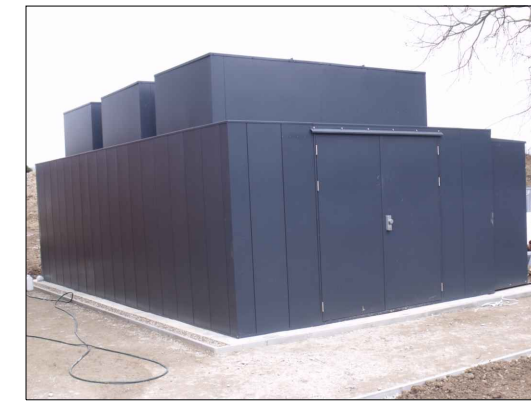
ASHP Acoustic Enclosure
