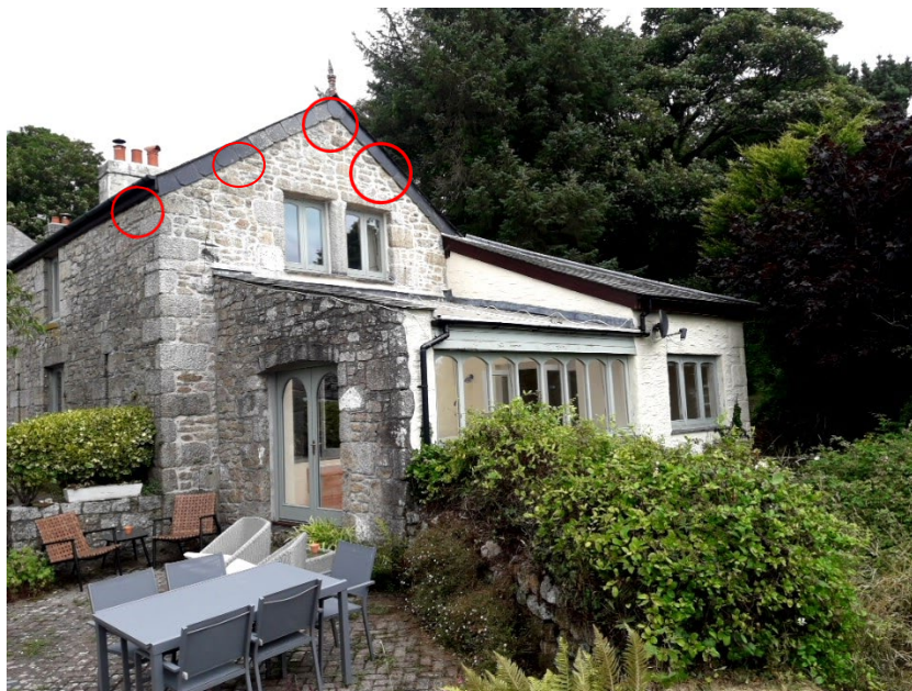
Figure 7. Southern elevation. Bat emergence points.
