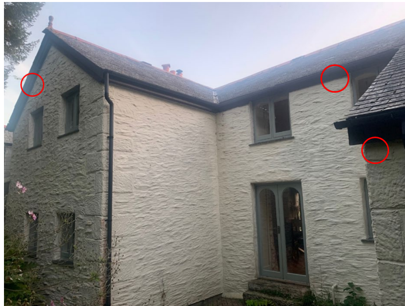
Figure 5. Bat emergence points, eastern elevation.
