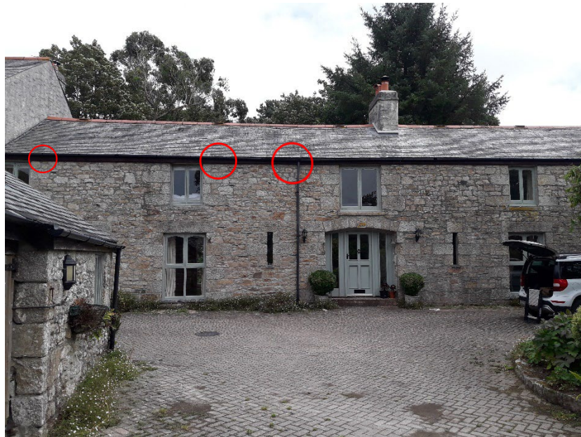
Figure 6. Western Elevation. Bat emergence points
