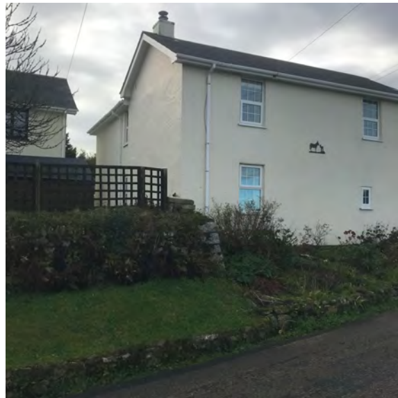
Services - BT overhead into dwelling:
