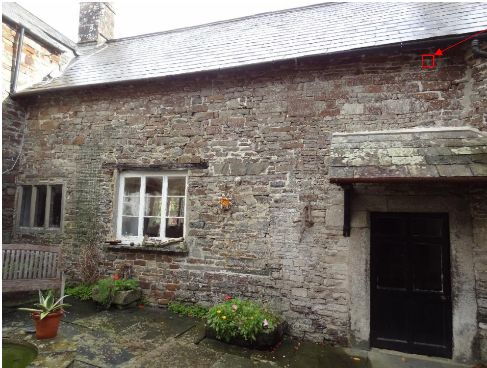
Figure 10 – Internal courtyard west elevation. Conservation vent grille with insect mesh to be installed and localised making good of stonework in lime putty mortar.
