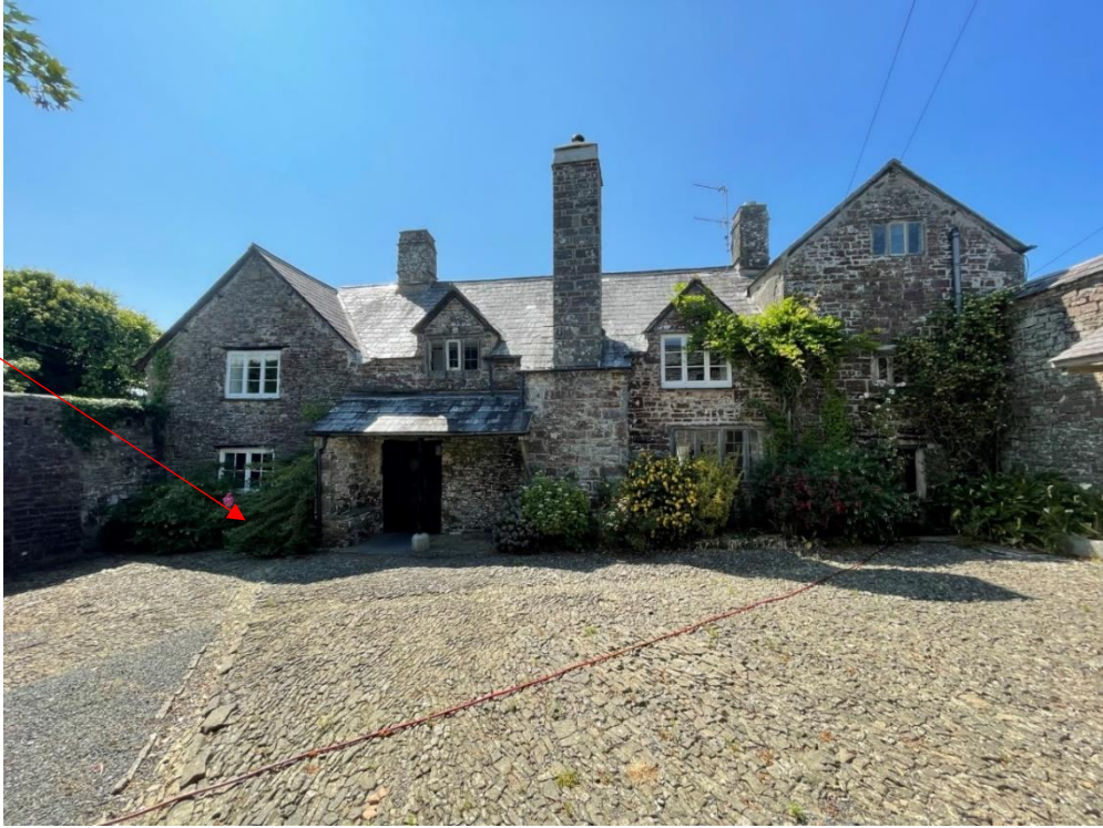
Figure 8 – East elevation. New soil pipe to exit at very low level to connect into existing underground soil pipe. Localised lifting of cobbles to enable installation of pipe branch, cobbles to be reset as existing.
