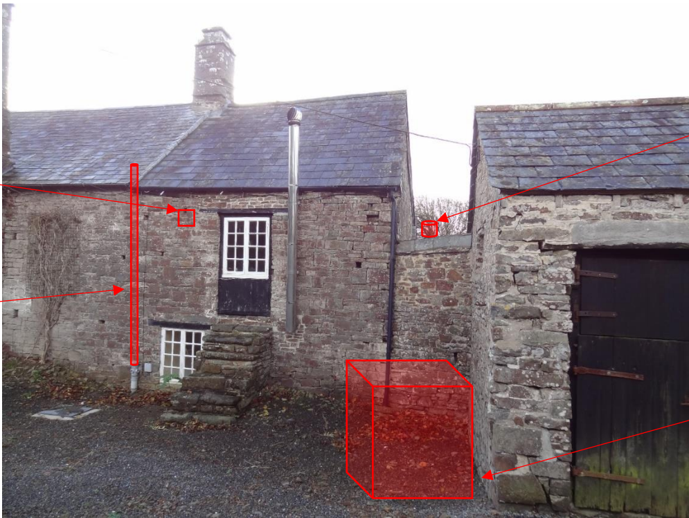
Figure 9 – North elevation. Conservation vent grille with insect mesh to be installed. New soil pipe connecting into existing stack and pipe replaced with cast iron pipework. Localised making good of stonework in lime putty mortar.
