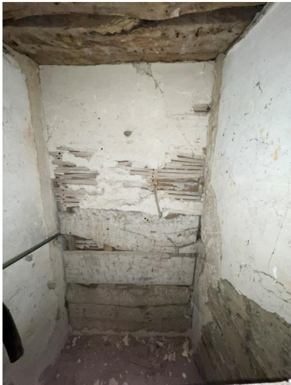
Figures 3-5 - Existing annexe bedroom to be converted into bathroom and opening to main Bedroom 1 to be reinstated. Photos showing timber plank and lath and plaster in-fill, timber lintels and plastered wall reveals, indicating historic opening, understood to have been blocked up in the 20th Century.
