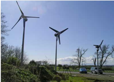
Wind Turbine Installation
