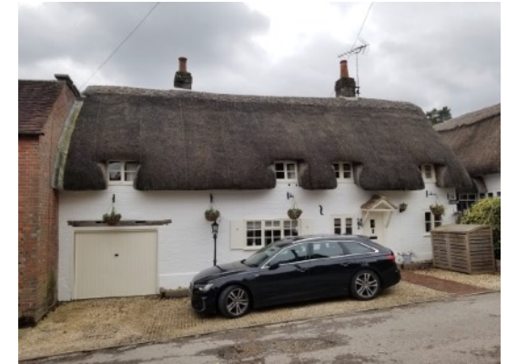
Existing East Facade showing Garage Door
