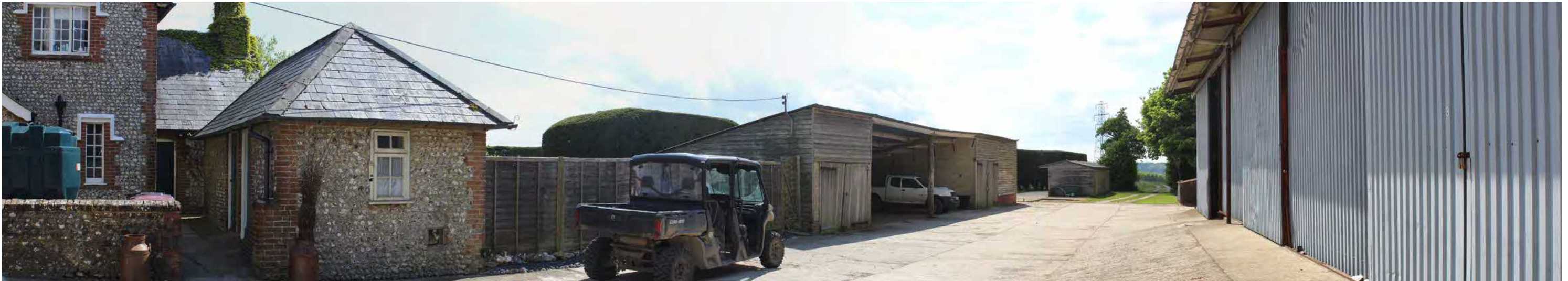
Photograph A. South westerly view across the farmyard in front of Colworth Farmhouse, showing the farmhouse's facade of knapped flint, framed within red brick quoins to the buildings corners and window edges and slate roof tiles. Timber featherboard fencing panels can be seen extending between the farmhouse and the barn proposed for replacement, which can be seen with sagging roofline, supported with a timber post, with timber clad, breeze block construction otherwise. A timber framed stable unit can be seen offset beyond. Beyond vegetation about the perimeter of the farmstead a glimpse of the far wooded skyline can be made, with a large metal electricity pylon overlying.
