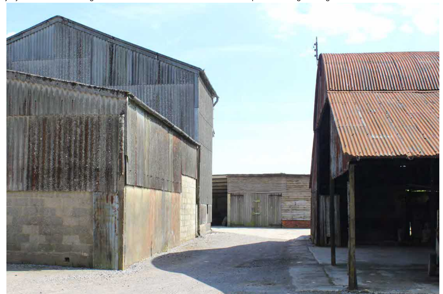
Photograph I. Southerly view. The roofline of the large agricultural buildings to the north of the farmstead can be seen. Modern building materials comprise of asbestos sheeting to roofs and facades of breezeblock wall construction. The earlier barn to the right of view comprises of corrugated iron roof, upon an iron frame. The barn proposed for replacement can be seen between the larger barns, with breezeblock and timber support poles to a sagging roof and timber cladding. Part of the fabric of the earlier farm building can be seen to the lower part of the barn to right comprising of red brick.
