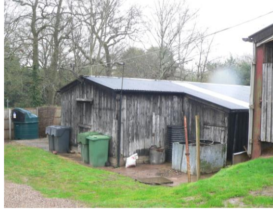
Barn on north side which will remain
