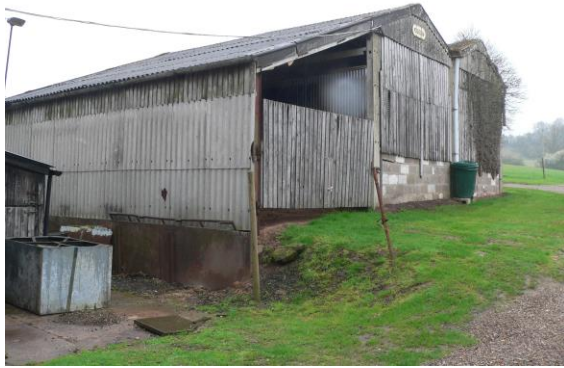
North west corner
