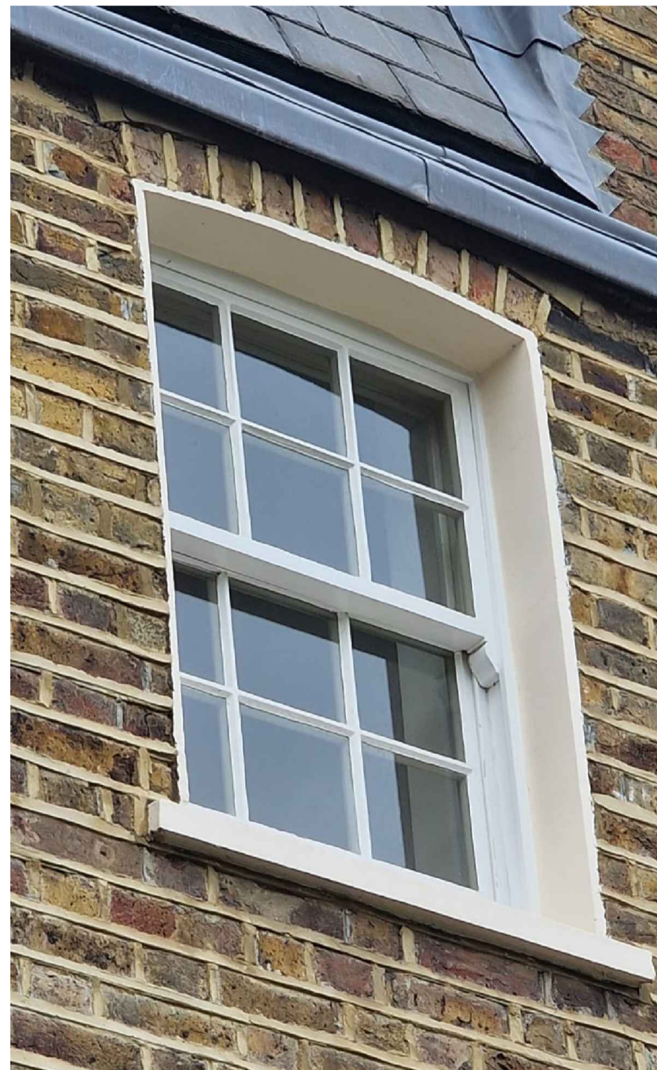
EXISTING PHOTO OF WINDOW 01
