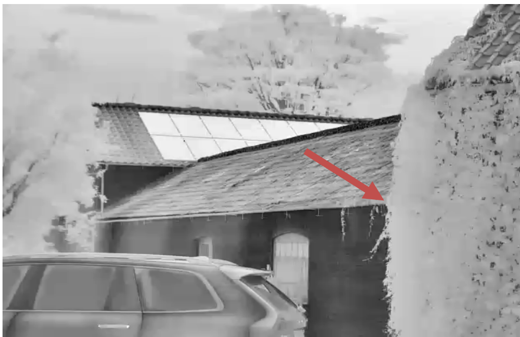
Photograph 7: Representative external view of Building 2 showing approximate bat emergence point
