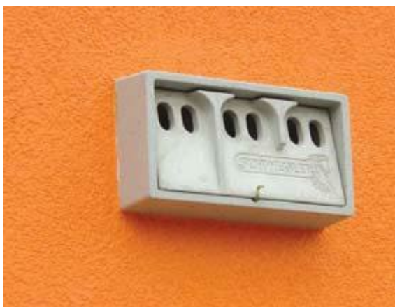
Photograph 8: Schwegler 1SP Bird Box Measures 245mm x 430mm x 200mm and weighs 13kgs.
