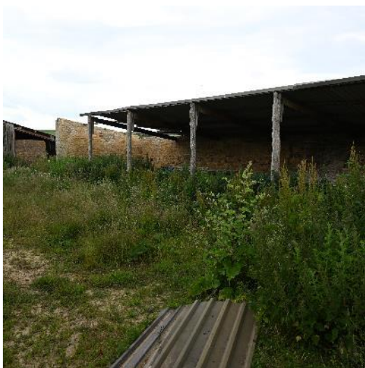
Image 10 Small open fronted sheds east of stone barn
