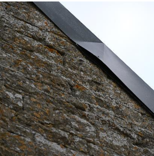
Image 4 PRF high up on roof fascia
