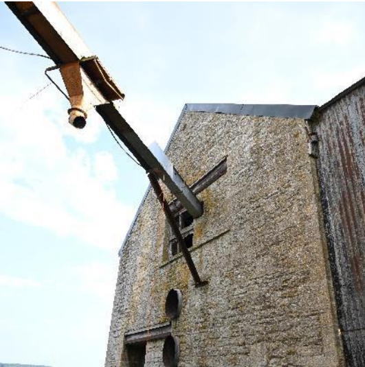
Image 3 Northern wall of large barn
