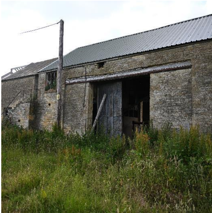
Image 1 Large stone built barn with double doors
