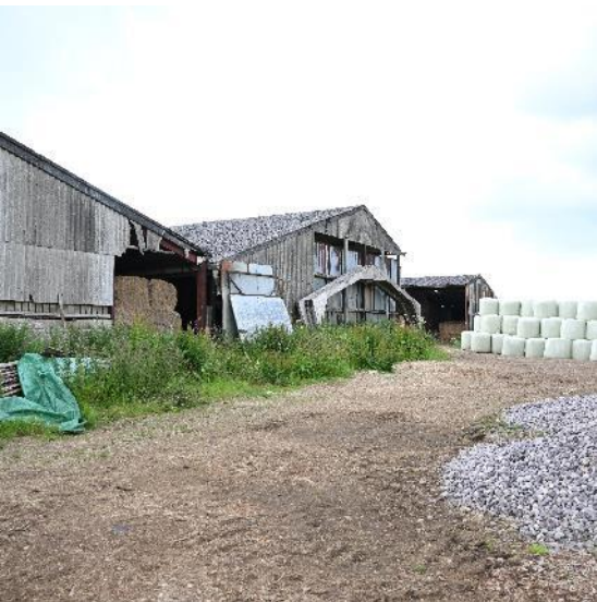
Image 5 Other barns on site
