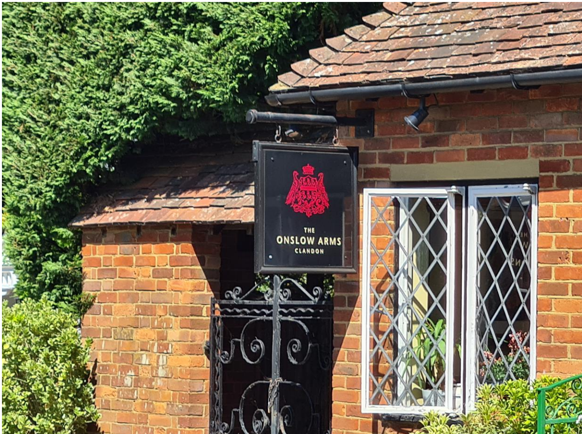
Photo H – Projection hanging sign on single storey extension. Approx. H700mm, Projection from wall 700mm. Spotlight illumination.
