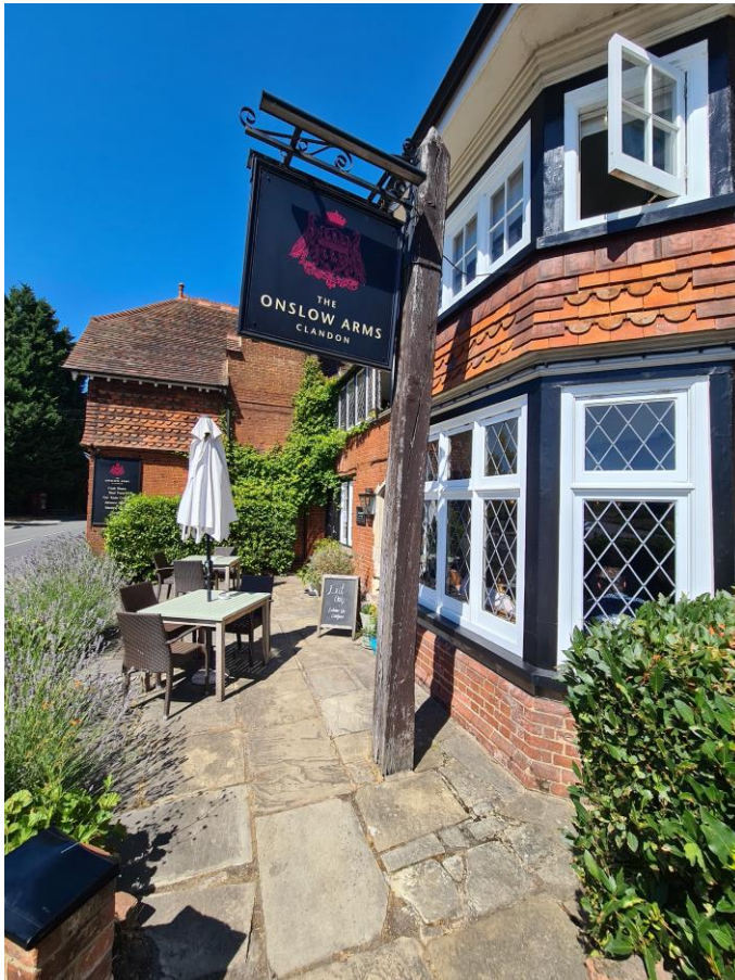
Photo B – Post swing sign to RHS of entrance. Timber post with signs of decay and suggest temporary support. Swing sign approx H1300mm, W1200mm. 2 x trough light illumination.
