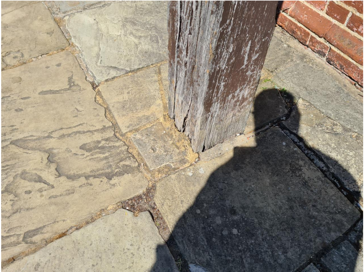
Photo C – Post base for swing sign showing signs of decay, recommend changing.
