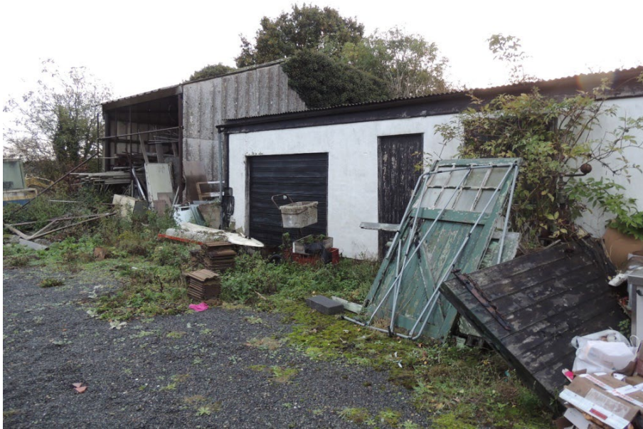
Photo 2: The existing sheds are unaffected by the project
