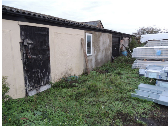
Photo 7: A building on the NW boundary is unaffected
