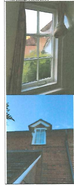
17 west passage (nearest porch)
