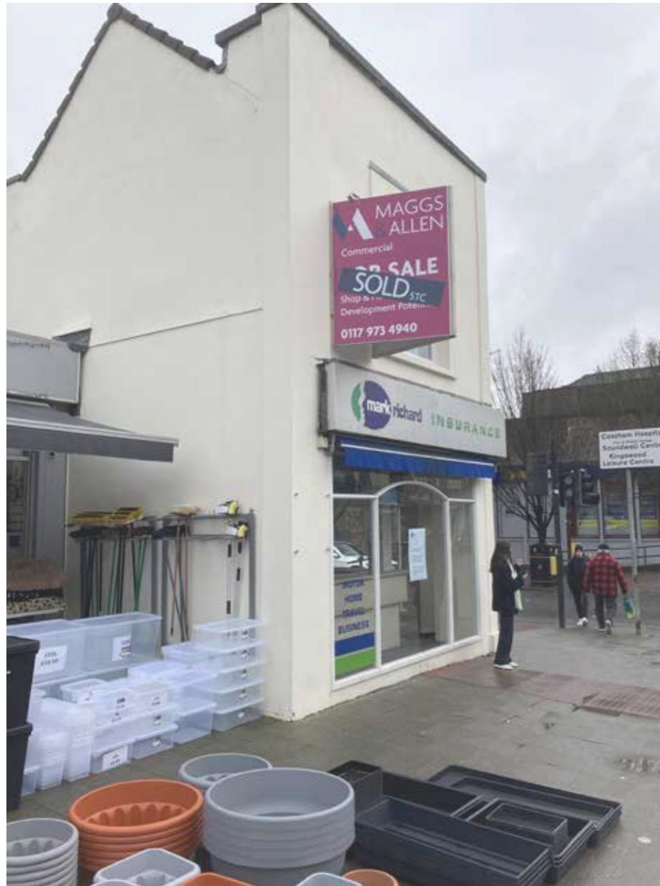
Street facing south elevation viewed from the High Street
