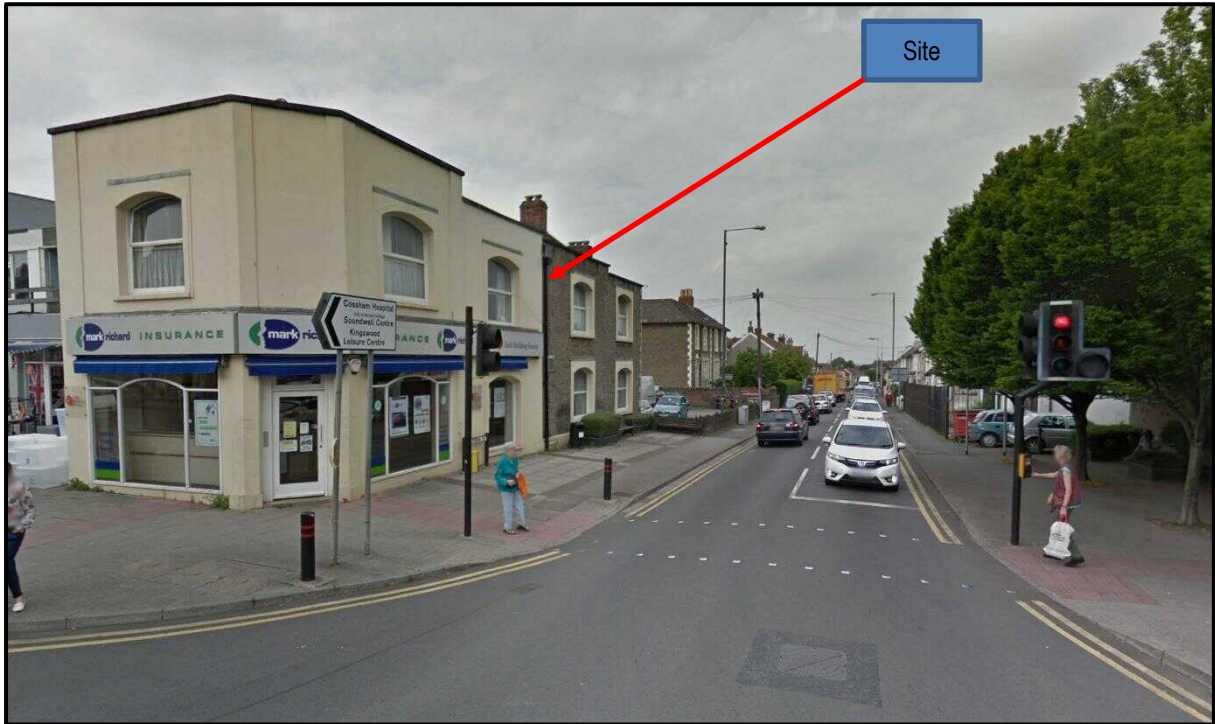
Figure 3 – General Site Photograph (taken from High Street Looking N)
