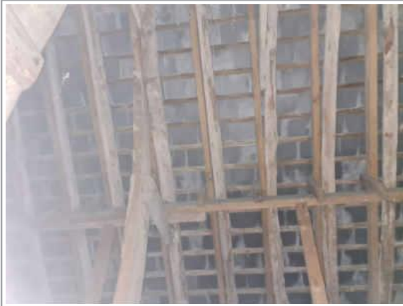
Single storey roof structure
