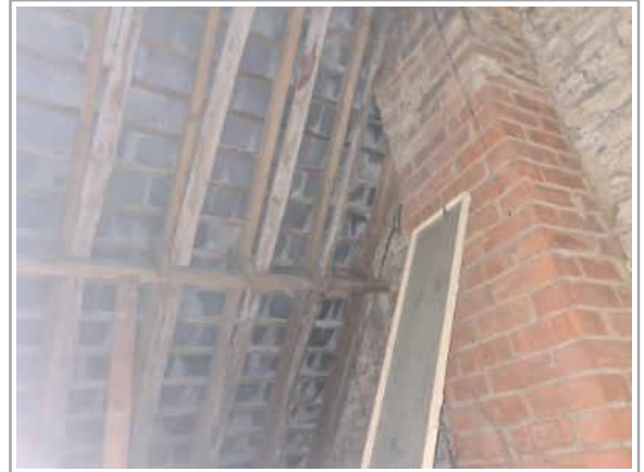
Single storey roof structure
