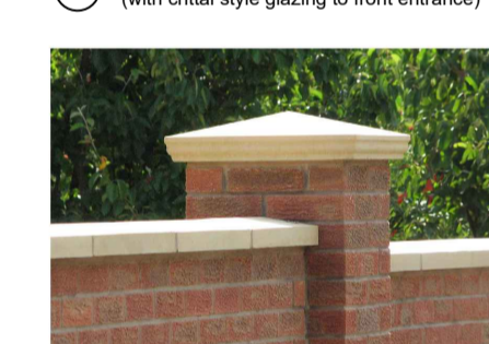
6 Facing brickwork retaining walls / piers with cast stone capping
