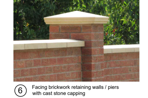
6 Facing brickwork retaining walls / piers with cast stone capping
