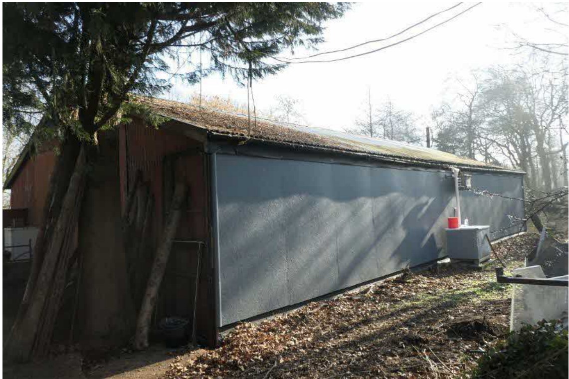
Photo 5, north and west aspects of building one, looking southeast.
