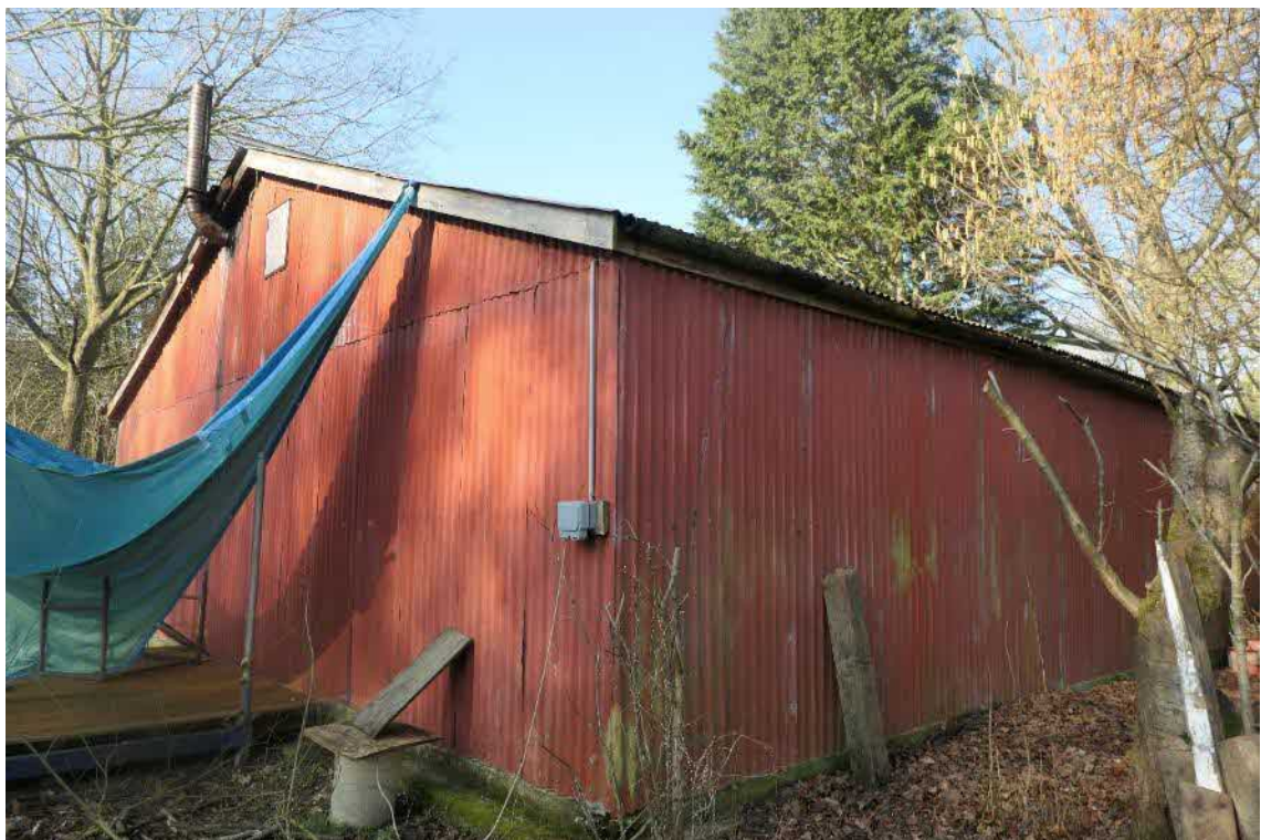
Photo 6, south and east aspects of building one, looking northwest.
