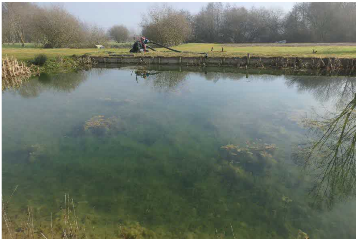
Photo 14, pond nine, looking east.
