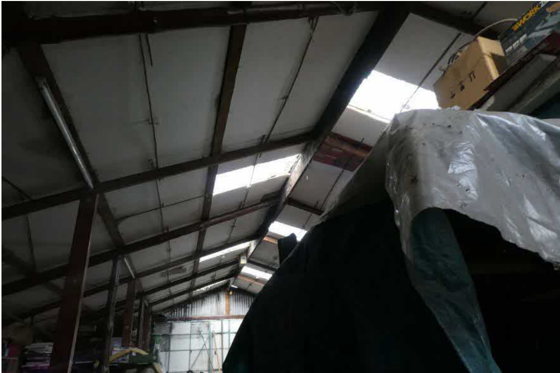
Photo 7, internal view of building one, looking south.
