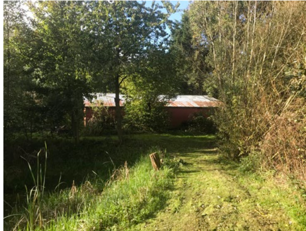
▲ Side elevation of the existing barn.
