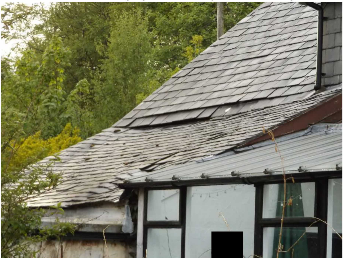
The defects in the roof where the garage and wood store join the main building
