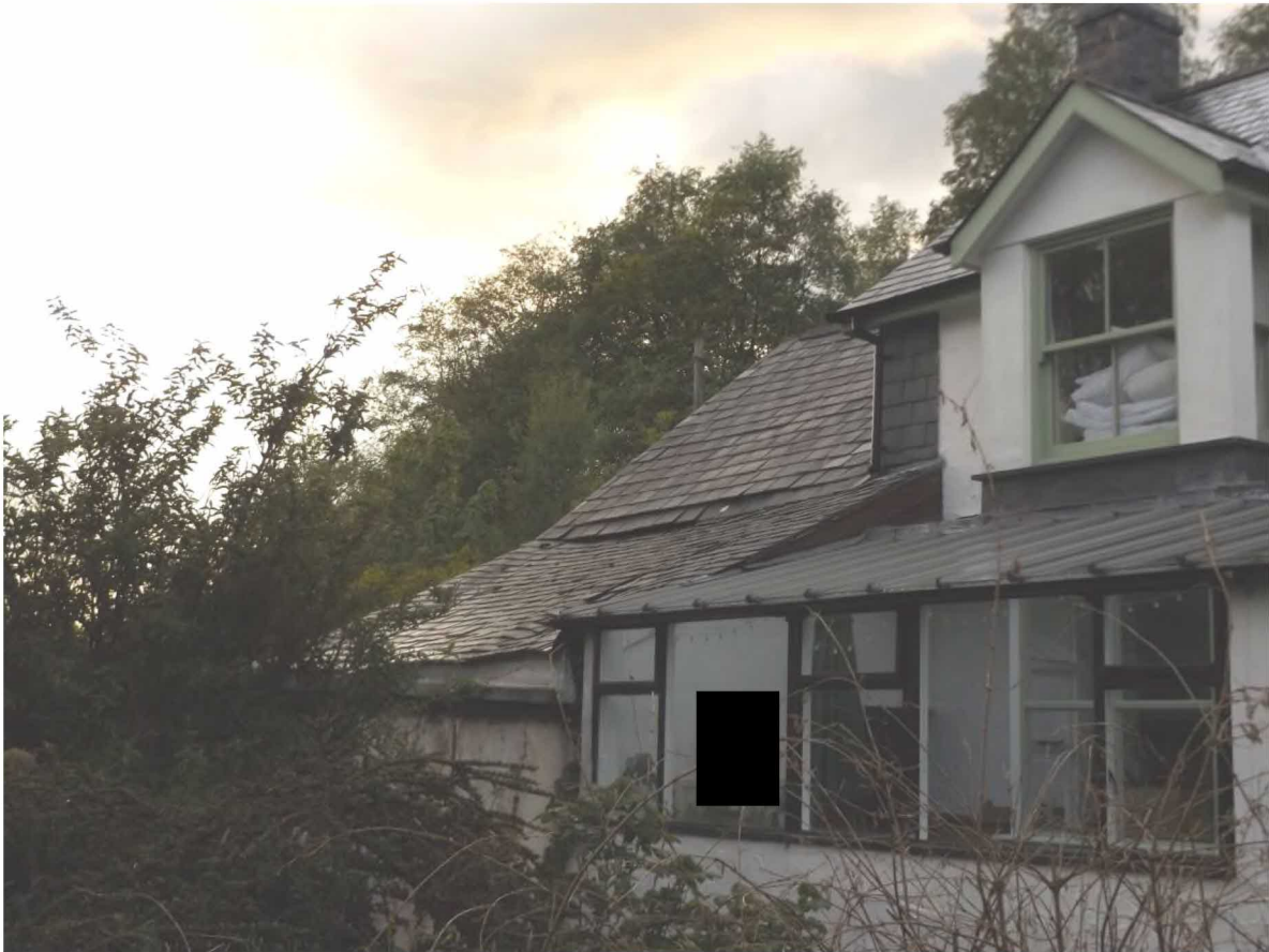
The defects in the roof where the garage and wood store join the main building
