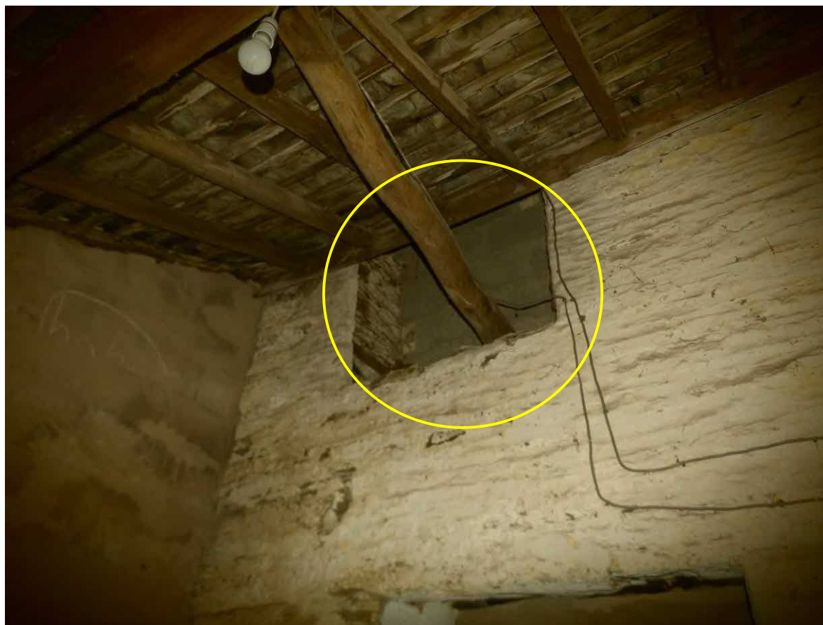
Figure 4: The recess created by sealing the original window
