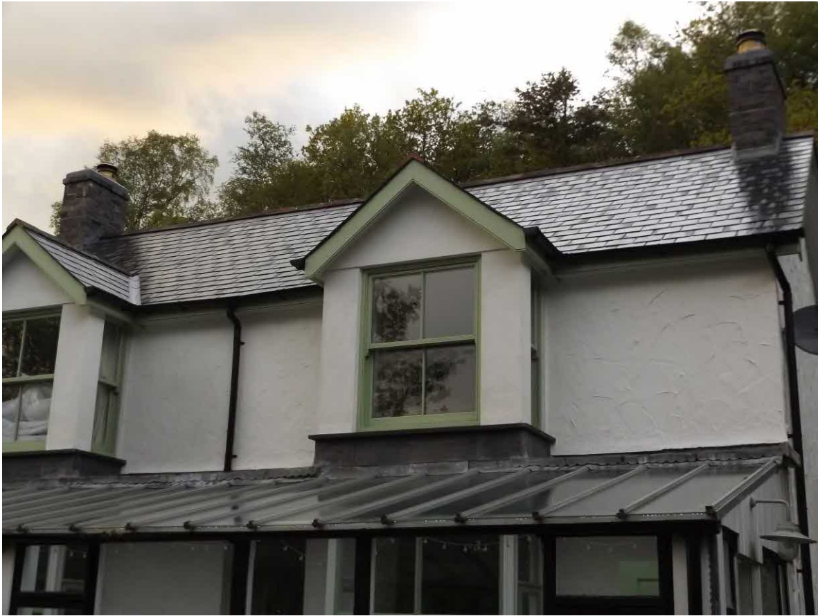
The new roof on the main part of the building
