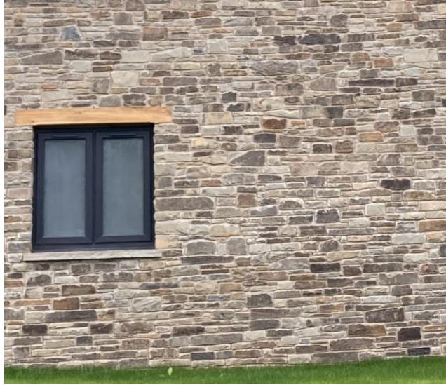
Figure 5: Details of 'Gladestry Quarry Cropped Walling Stone' Masonry Stonework.
