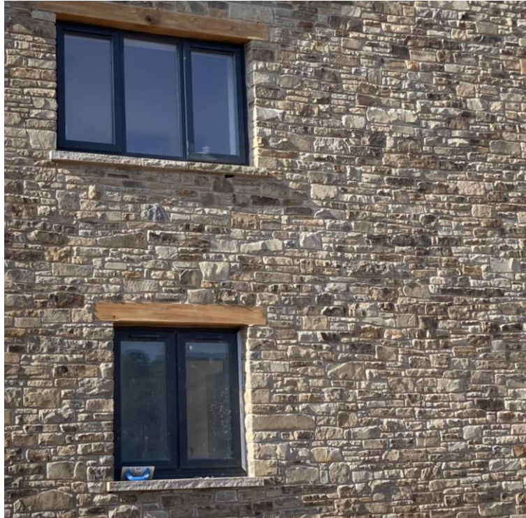
Figure 6: Details of 'Gladestry Quarry Cropped Walling Stone' Masonry Stonework.
