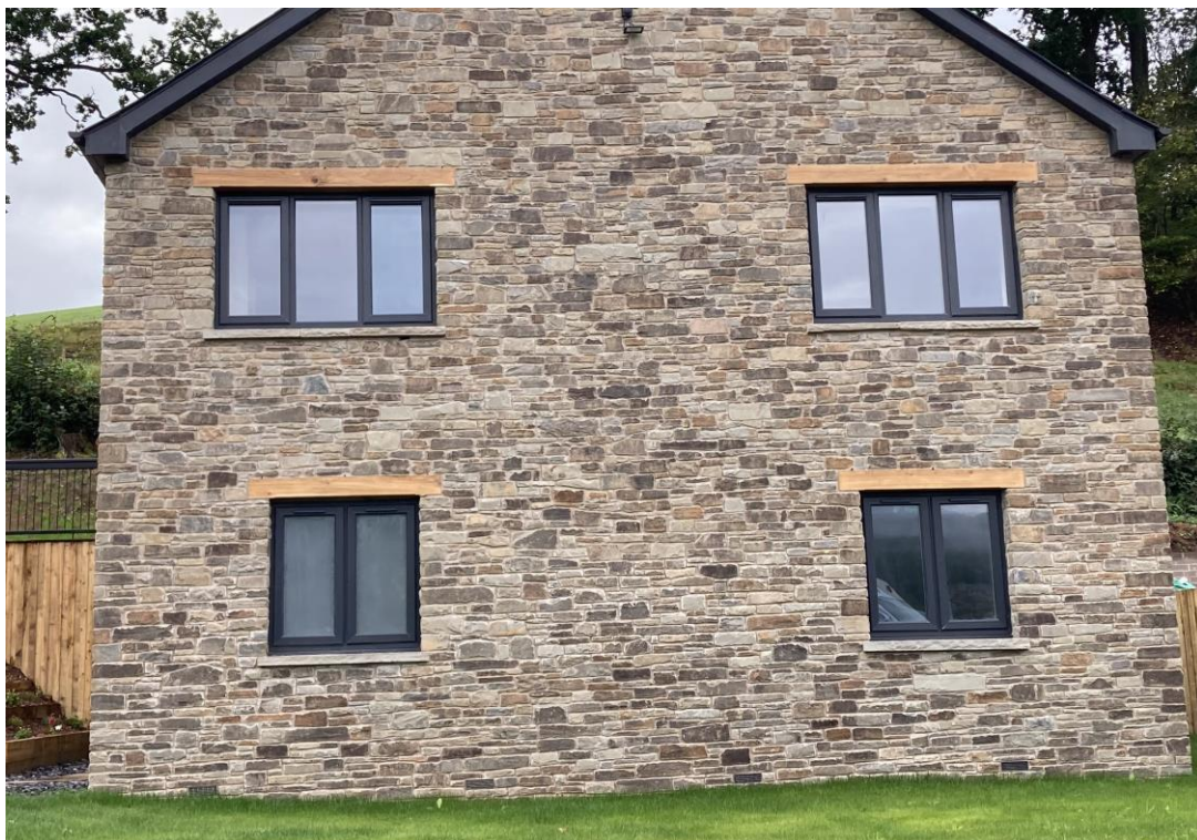
Figure 1: Details of ‘Gladestry Quarry Cropped Walling Stone’ Masonry Stonework.
