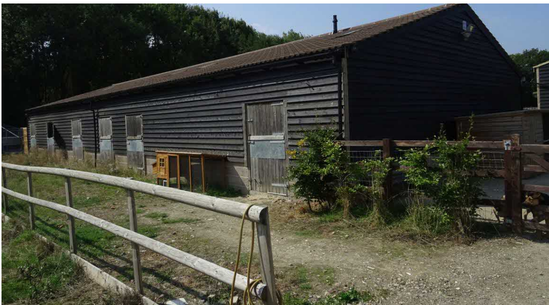
Photograph 10. Path to Door 04/09/2018
