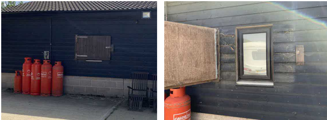
Photographs 12 & 13. Spare Room Window
