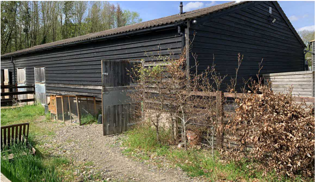
Photograph 11. Path to Door 03/05/2023
