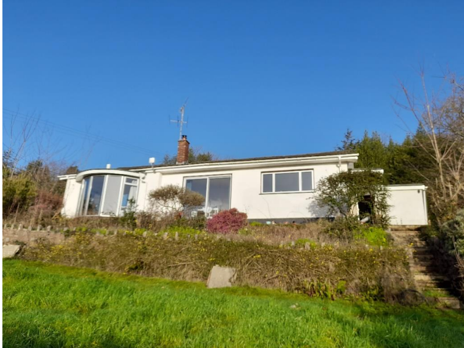
Plate 4 – Southern elevation of the bungalow
