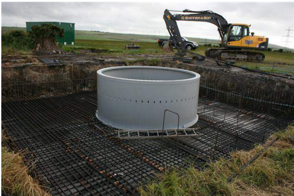
Figure 5: Example of Turbine Concrete Base Preparation
