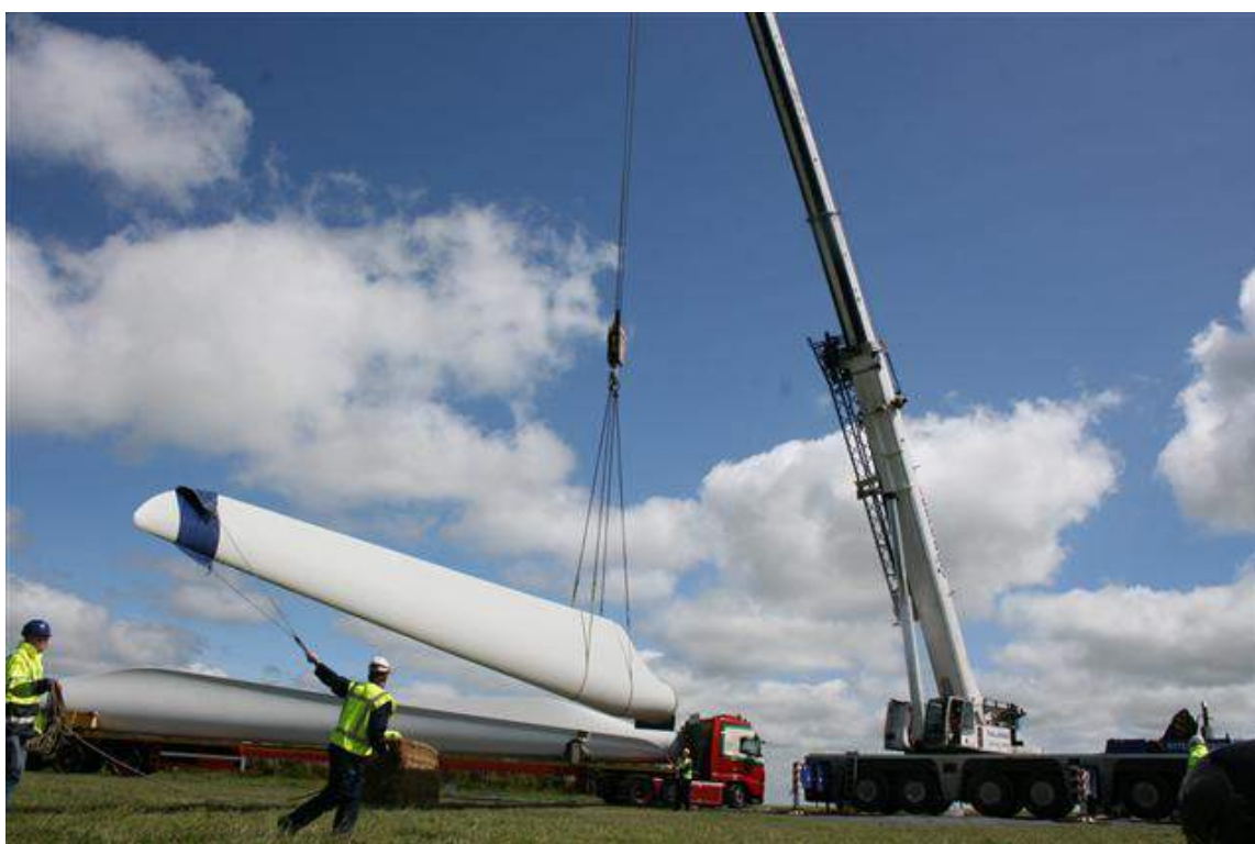
Figure 6: Use of Telescopic Crane to assemble Turbine
