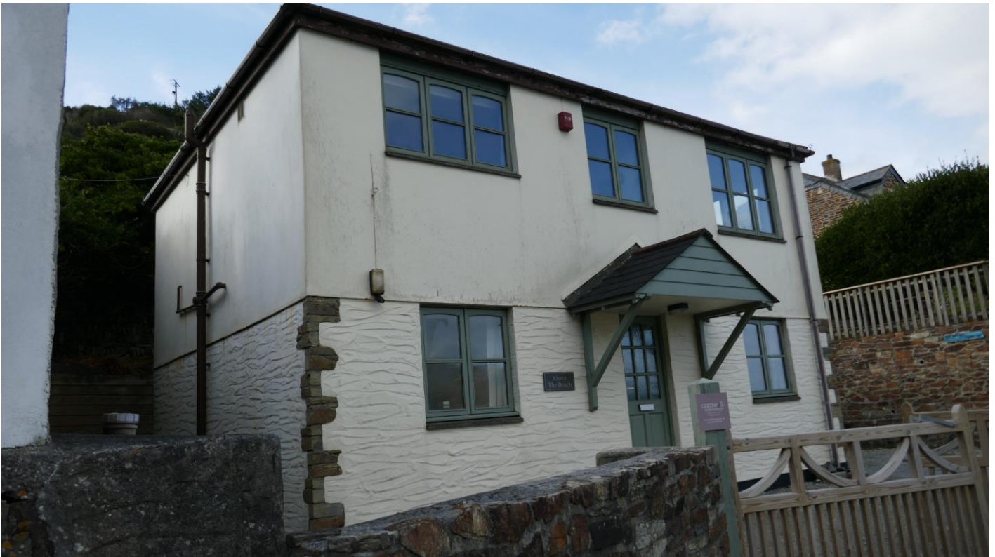
Figure 1. Southern and eastern elevations of the building.
