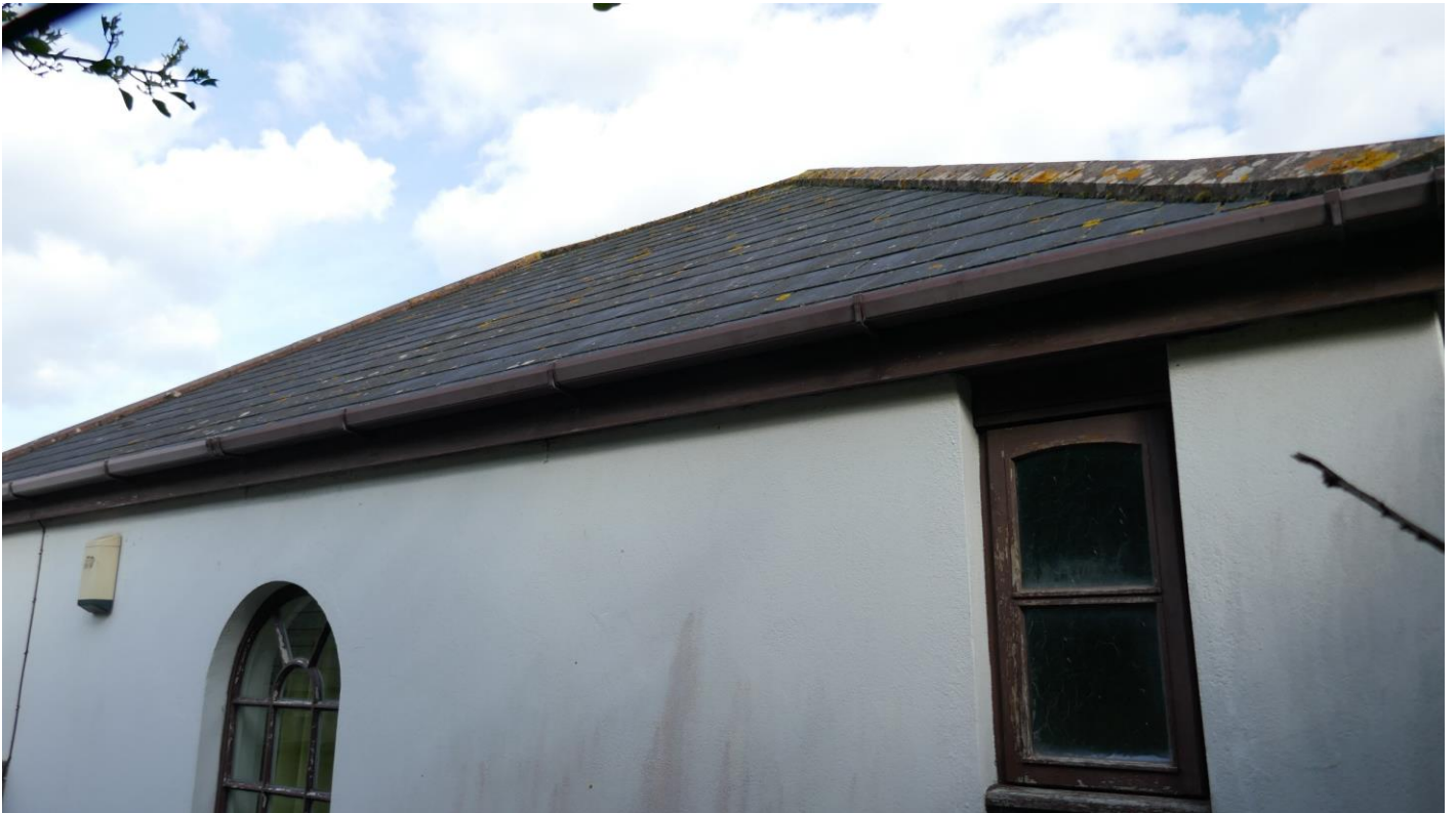
Figure 3. Roof on western aspect of the building.
