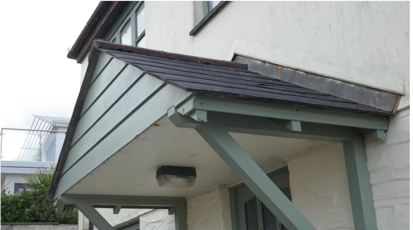
Figure 5. Porch above entrance door on eastern aspect of the building.
