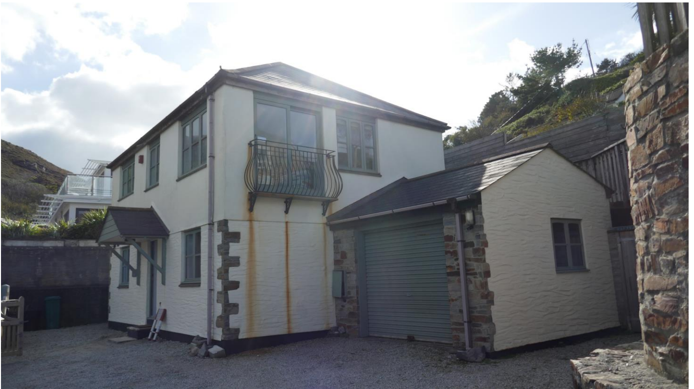
Figure 4. Northern and eastern aspect of the building with built-on garage.
