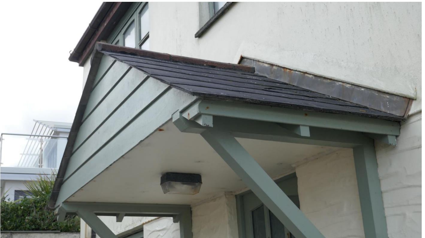
Figure 5. Porch above entrance door on eastern aspect of the building (October 2022).
