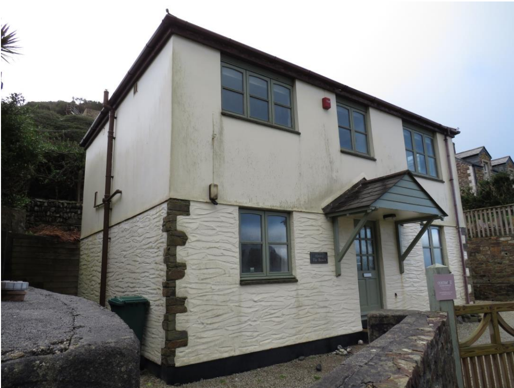
Figure 1. Southern and eastern elevations of the building, November 2023.
