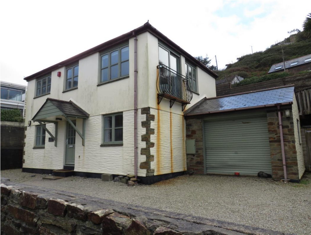
Figure 4. Northern and eastern aspect of the building with built-on garage (November 2023).
