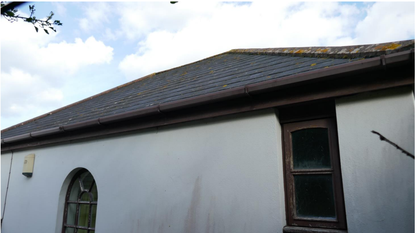
Figure 3. Roof on western aspect of the building (October 2022).
