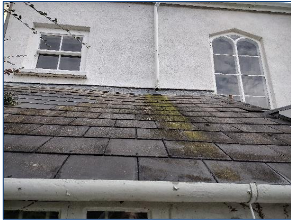
Tight fitting tiles with single raised tile
