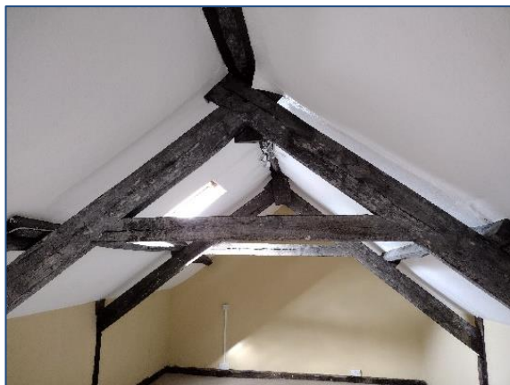
Interior (loft space)
