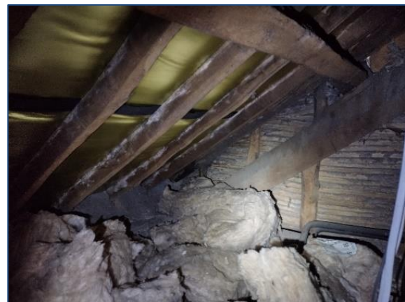
Interior (eave cupboard)
