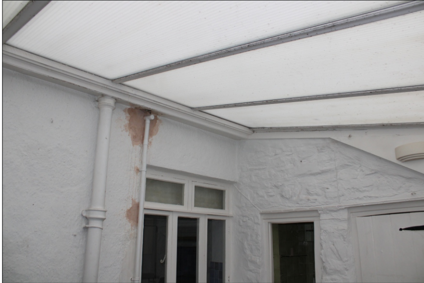
Plate 11: View of roof in the conservatory, looking east
