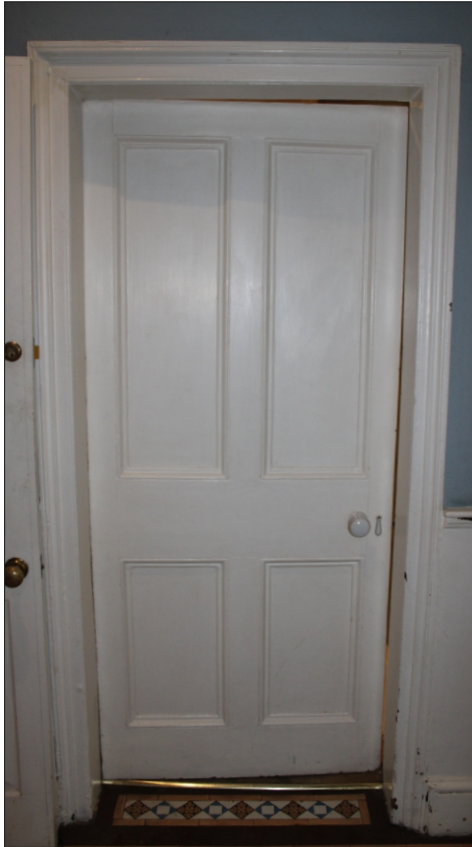
Plate 7: 19th-century four-panel door into southeast reception room, looking southeast
