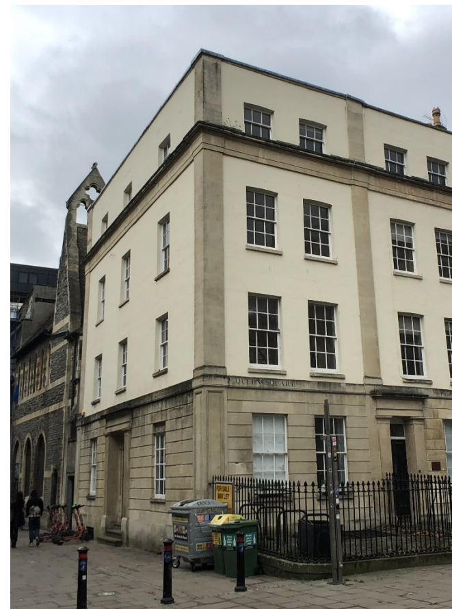
Photo 1. No. 46 Queen Square prior to conversion from office into a 9-bed house in multiple occupation.
