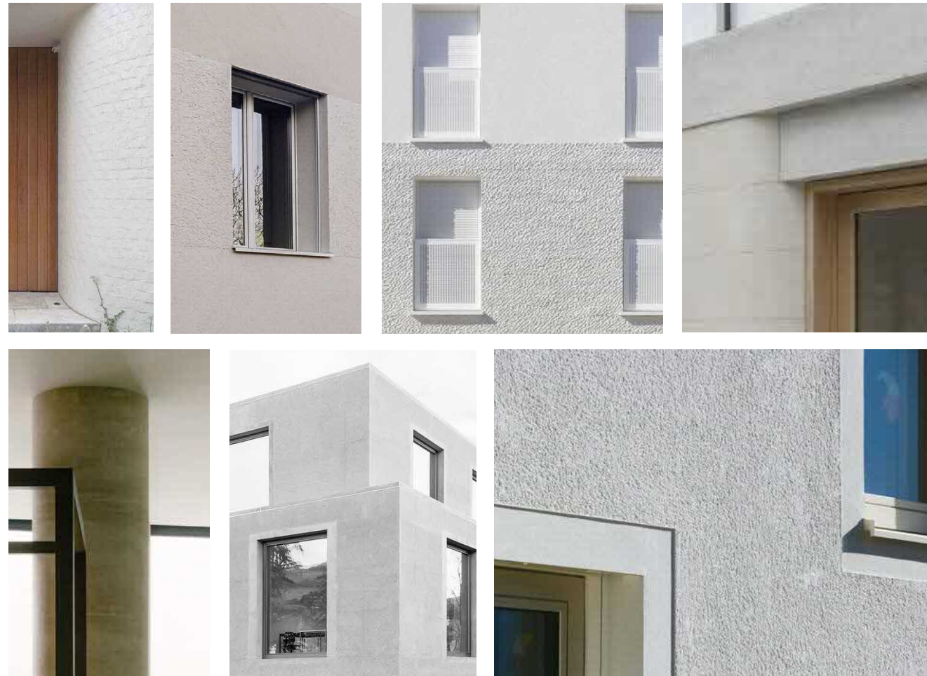
Visual references: Example projects using textured and smooth render to create relief and definition to window openings and entrances. The rendered column is proposed to celebrate the curved language and modernist character of the street
