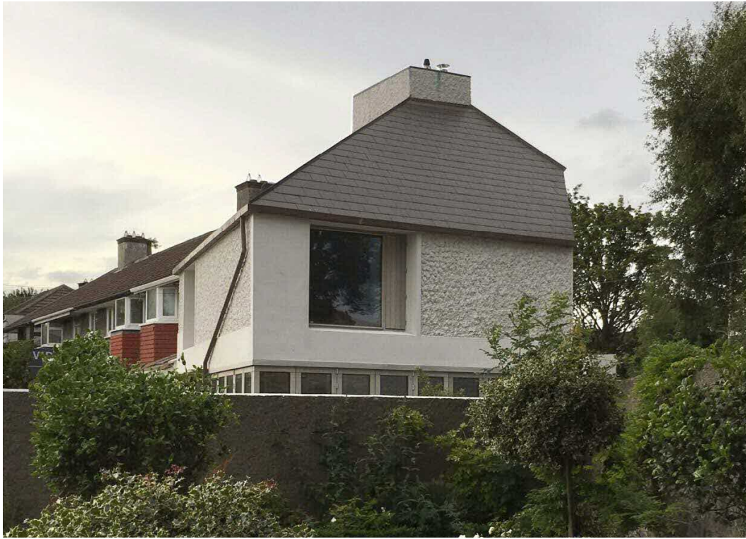
Visual reference: Example project using textured and smooth render as well as tiles, chimney and corner glazing to achieve a contemporary take on suburban character
