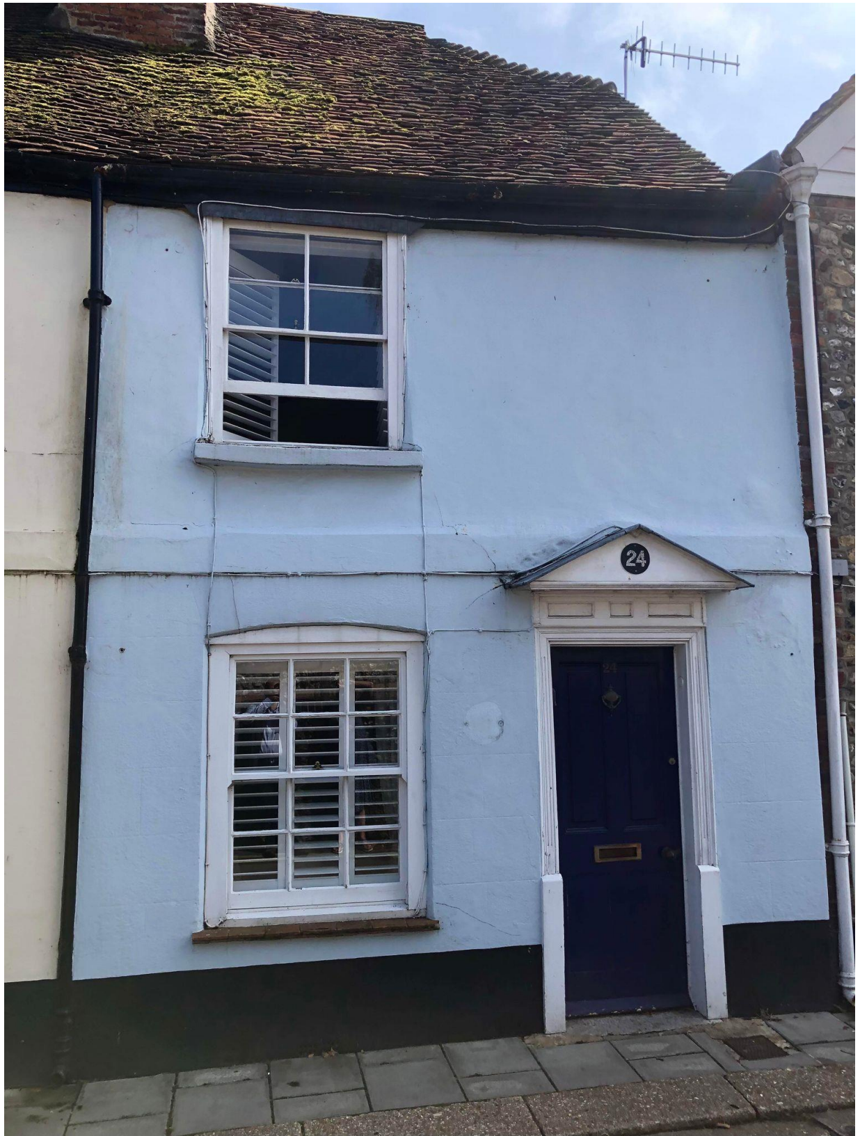
Fig 5: The principal elevation of 24 North Street as seen from the city walls. The building was refronted in the 19 th Century and adopted a Georgian architectural style. The building would not require any structural changes as a result of the proposals.
