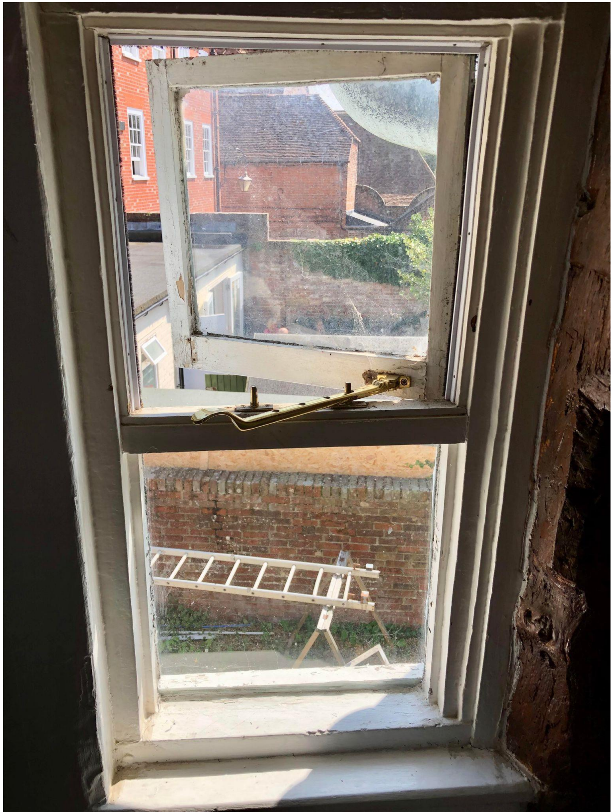
Fig 6: The existing stair window dates from the 20 th Century and does not constitute historic fabric. The proposed sash design would represent an improvement over existing, enhancing the buildings significance.
