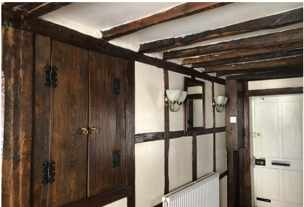
Fig 2: The principal reception room of 24 North Walls on the ground floor showing the timber framing construction of the building. The historic fabric of the Grade II listed building would not be harmed by the proposals.
