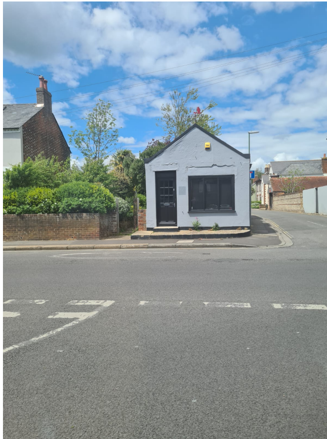
Figure 1. South Elevation as viewed from Oving Road
