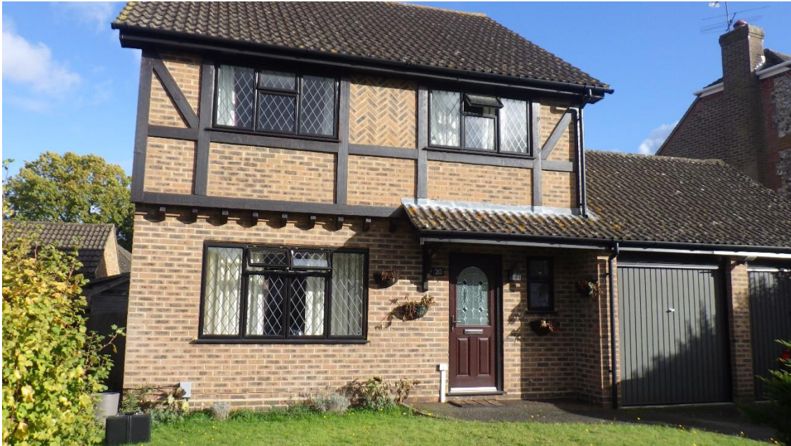
Front (West) Elevation of the property
