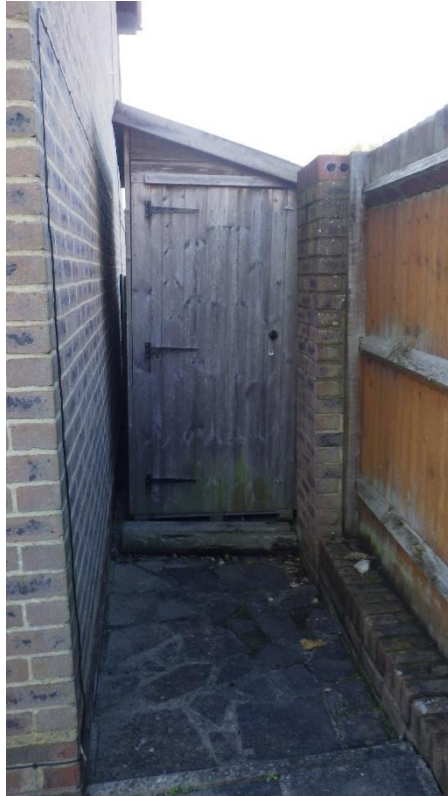
Rear (East) Elevation of existing shed
