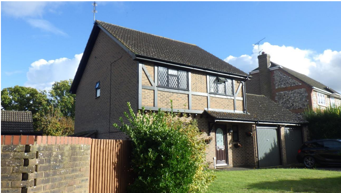
Wider view of the north side of the property
