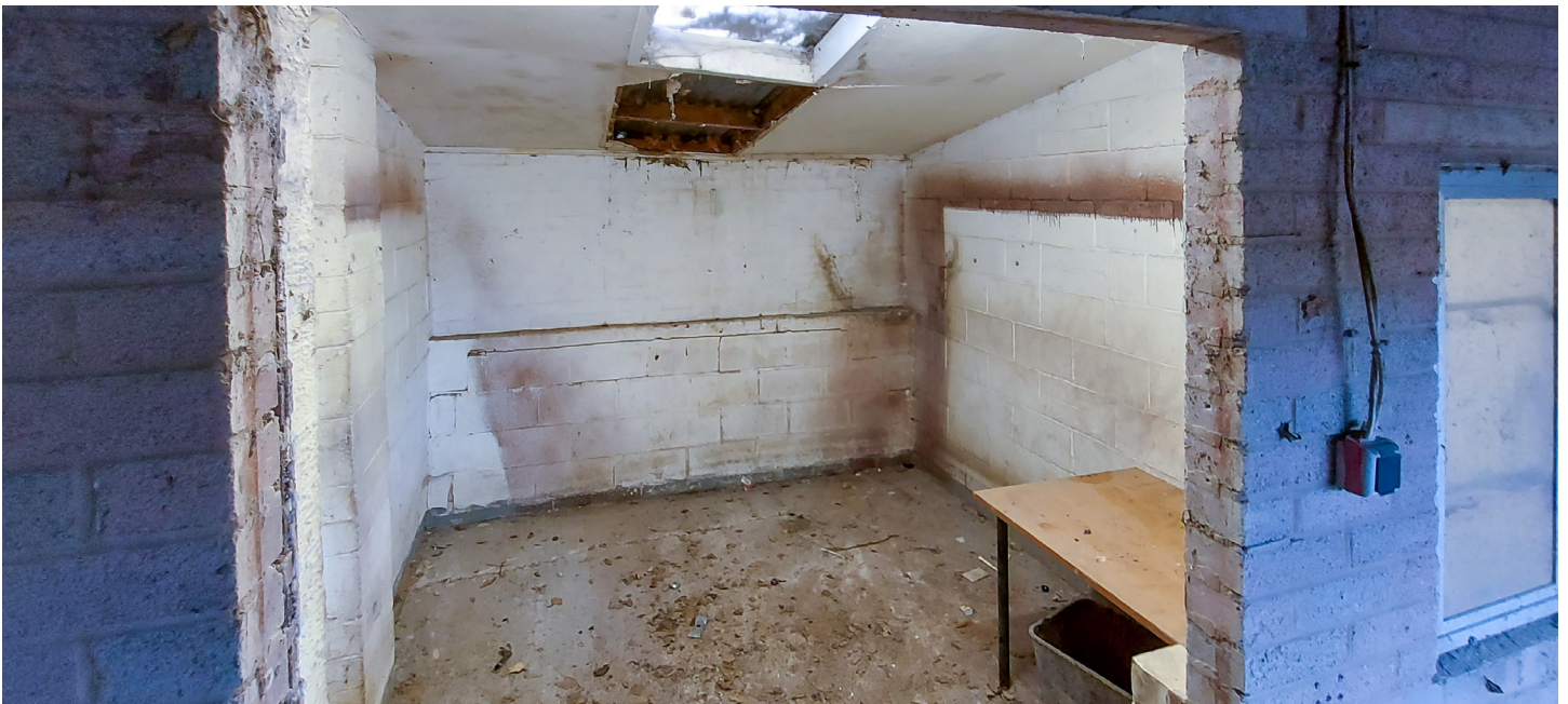
Interior photographs of Croppings Green Wood Stables
