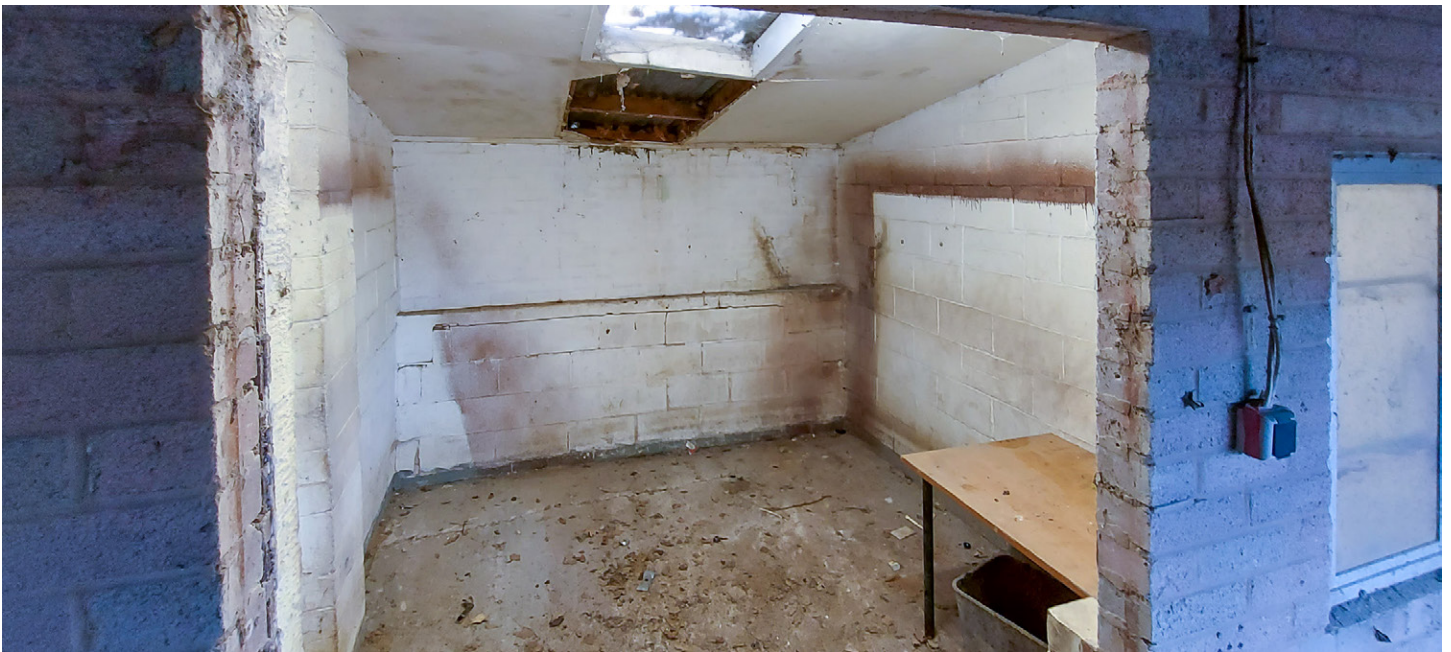
Interior photographs of Croppings Green Wood Stables
