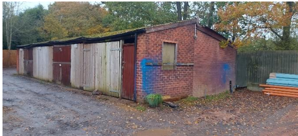
Plate 2: Showing a typical view of the Stable Block. Photograph looking south.
