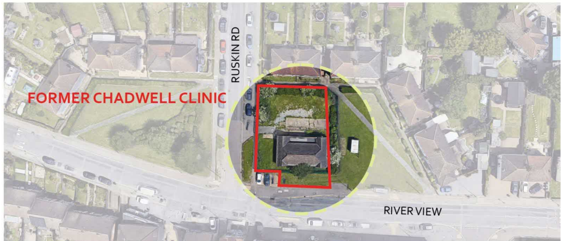
Fig.1 Ariel Photo of Site
