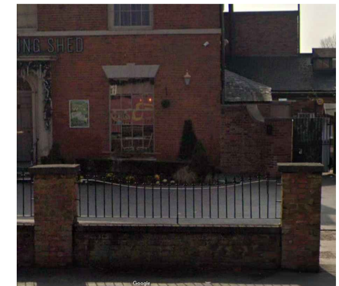
IMAGES 6 - EXISTING WALL AND FENCE
