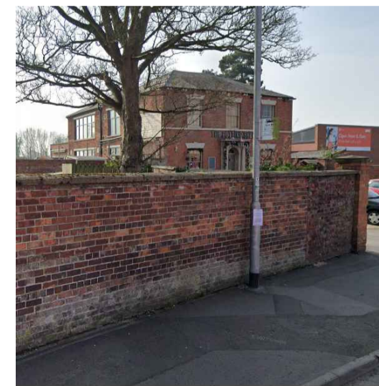
IMAGES 5 - EXISTING WALL
