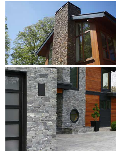
Stone Surround to entrance and chimney
