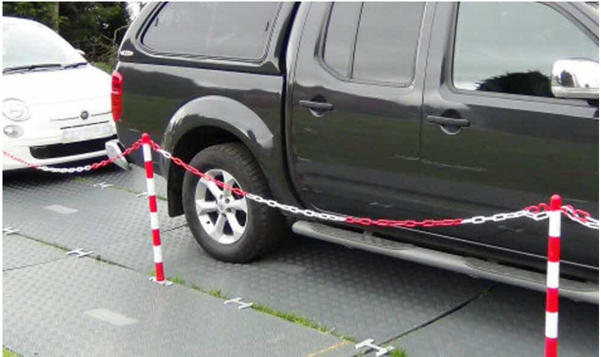
Fig. 3 Ground Guards Lite Track provide a suitable surface for vehicles and light construction plant over the cellular confinement area
